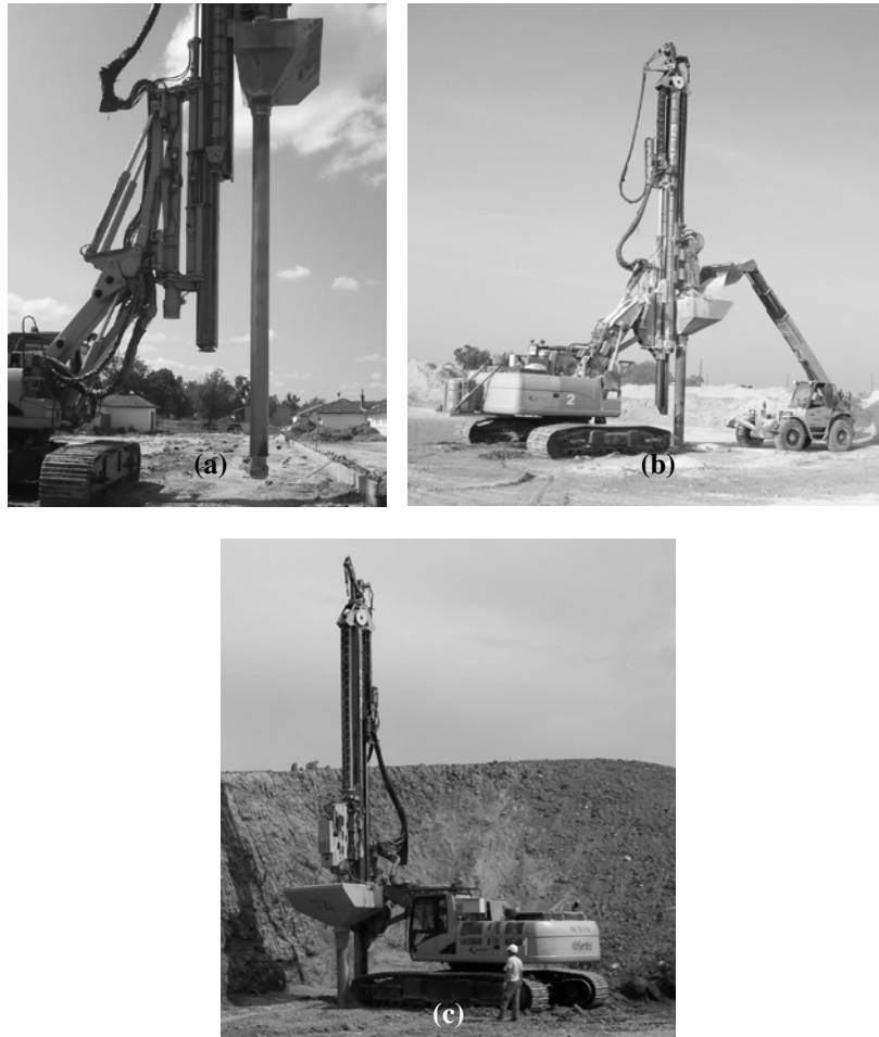
Figure 1. The construction of Impact Rammed Aggregate Piers.
