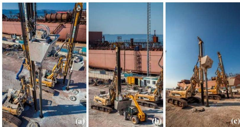
**Figure 2.** The construction of Impact RAPs
