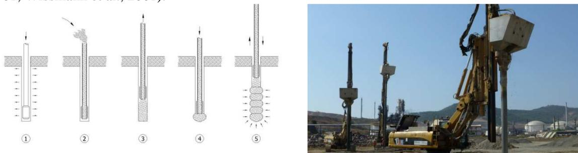
Figure 3. Construction methodology of Impact Pier® and a view from the field construction
